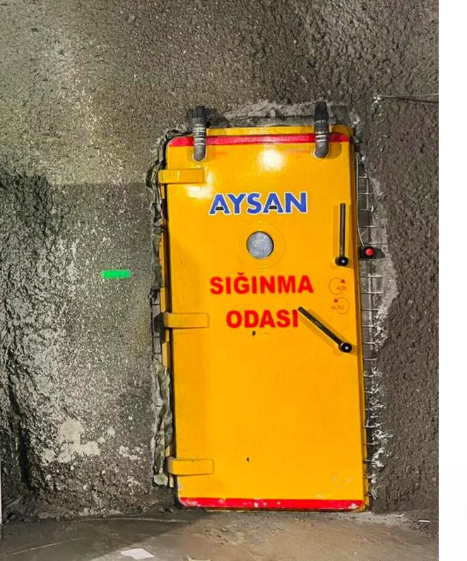
Permanent Refuge Chambers are formed by sealing concrete rooms formed in mines. In terms of cost-effectiveness, this system offers the best solution for large numbers of people underground at a time.
